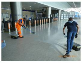
**Step 4:** Application of the Recoat Floor, extremely hard wearing Anti-Slip Coating.
