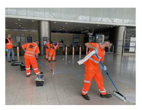
**Step 3:** Application Recoat Multi Primer Clear, universal, waterborne, clear primer which adheres exceptionally well to most substrates
