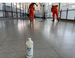
**Step 2:** Application of the Recoat Bonding Cleaner to ensure optimal adhesion to the terrazzo tiles without abrading.
