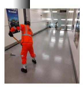
Figure 1 Application Recoat Anti Slip Topcoat in escalator area
